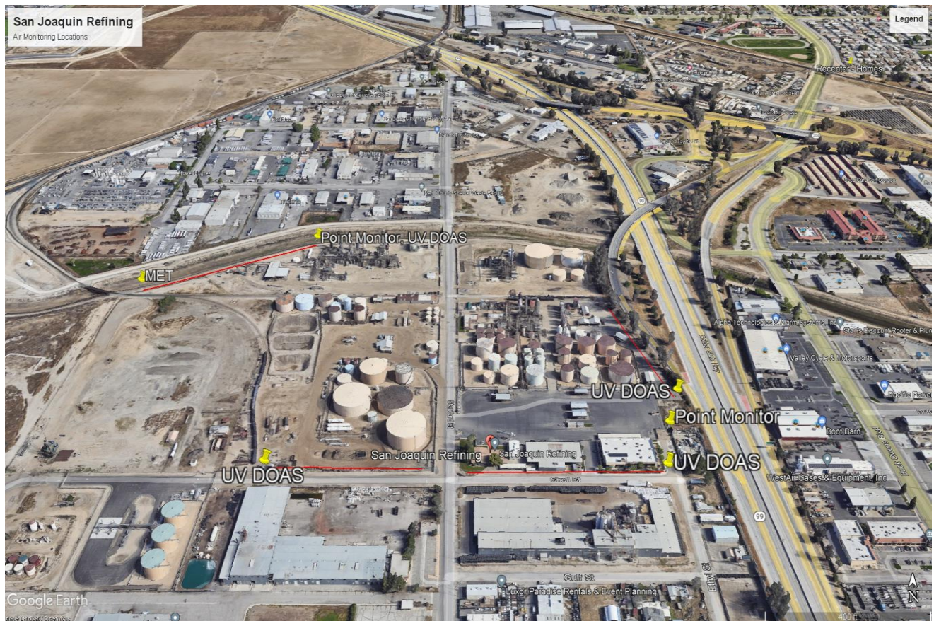
Figure 2.1 - Map of Fence line Monitoring (red lines are UV DOAS, point monitor locations are noted )
