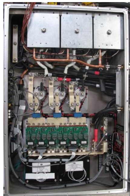
Figure 9. Interior of ICU.
