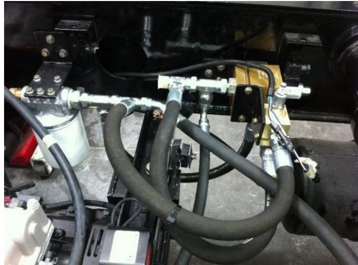
Figure 18. Hydraulic plumbing in the IKEA tractor.
